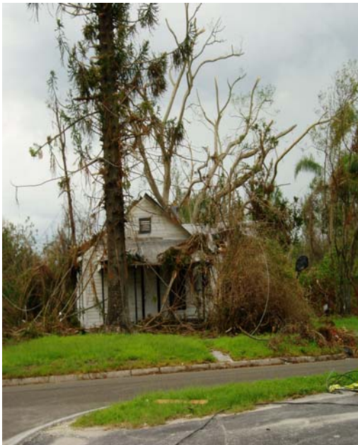
Hardee County house after hurricane.
